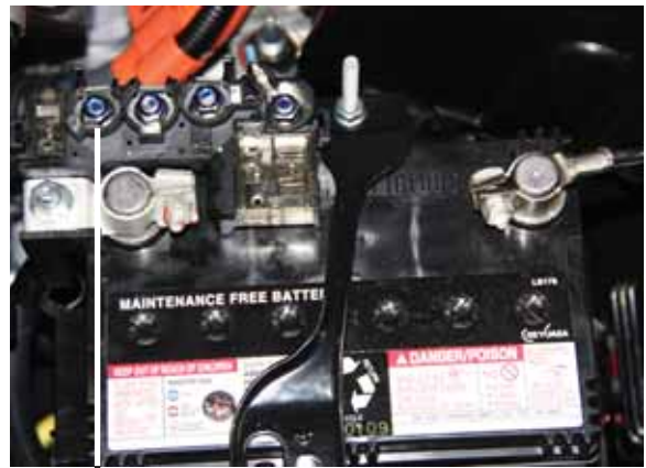
DC to DC Converter Cable Connection
