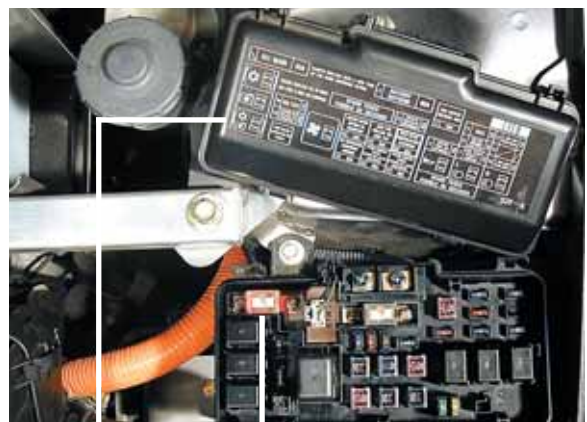
Fuse Box Cover
